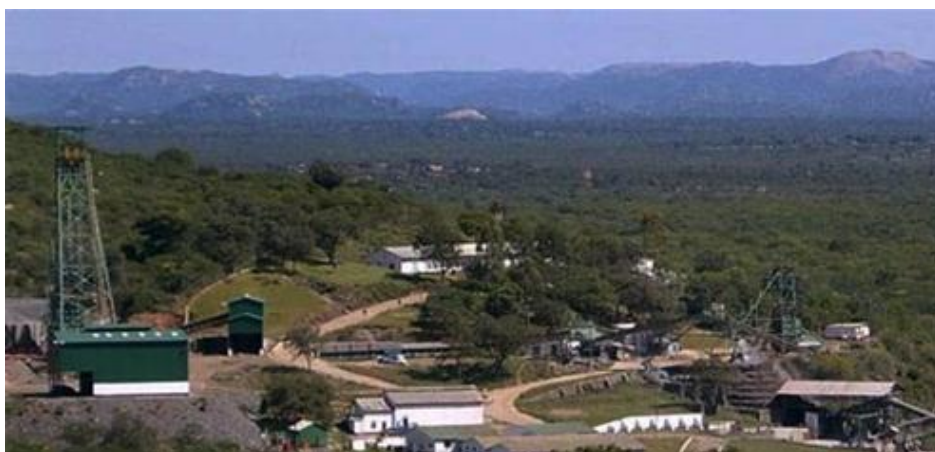
Figure 6: View of Blanket Mine
