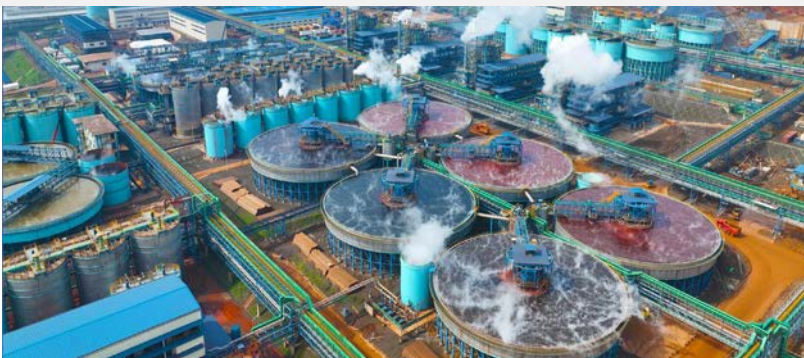
Huayue HPAL Project
