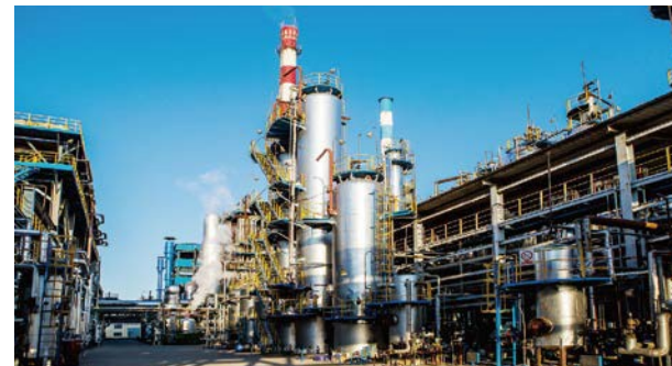
Cobalt, Copper Smelter
