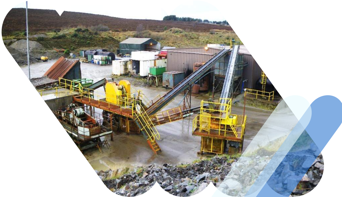
Processing plant showing jaw (left) and cone crusher (right)
