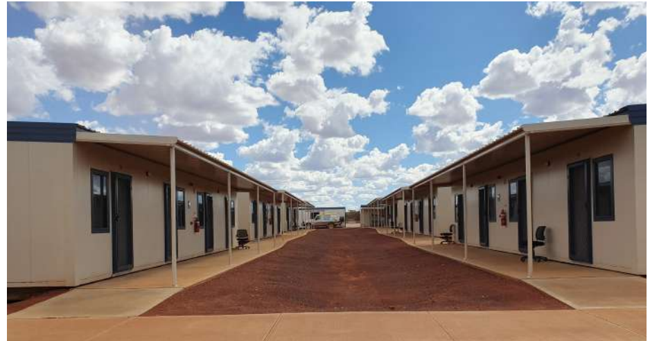
Stage 1 of commissioned permanent camp
