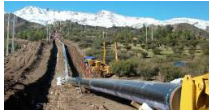
COPPER CONCENTRATE SLURRY PIPELINE 2
