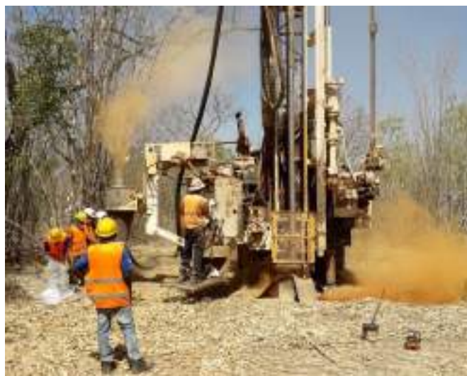
Operating RC Drill Rig
