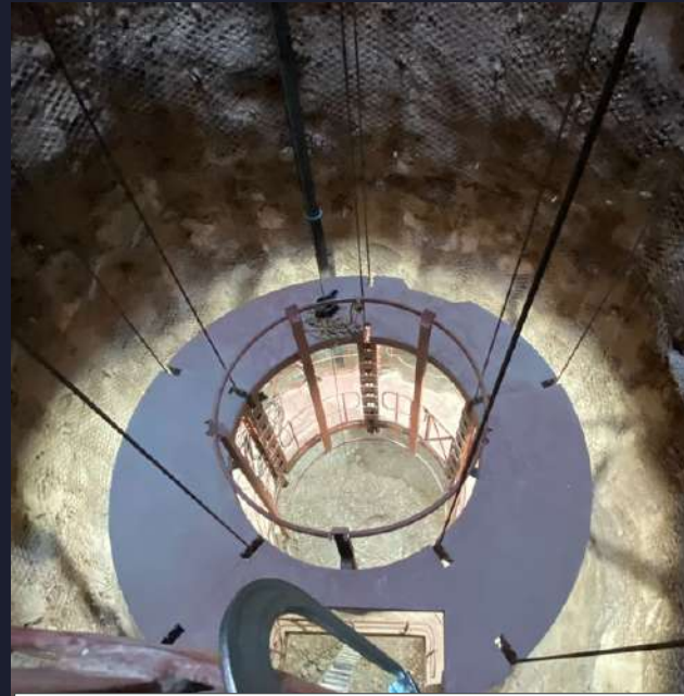
Vent Shaft Pre-sink stage view from above
