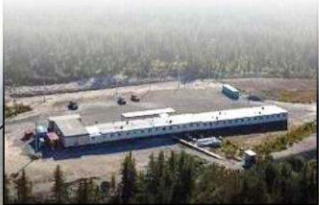
Initial Construction Starter Camp *installed septic
