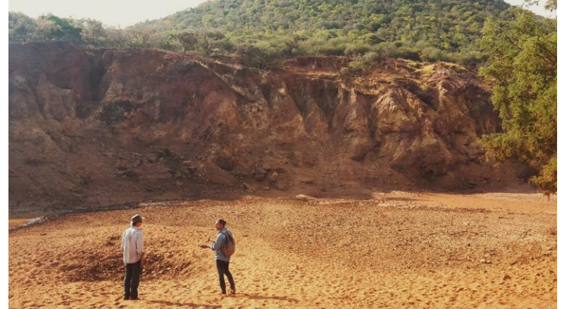
Source of DSO material - rehabilitation work on Otse pits and old stockpiles from K.Hill
