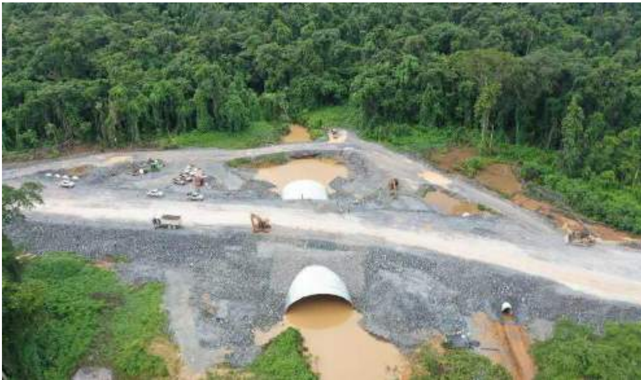
Mindrinetti Bridge – Complete
