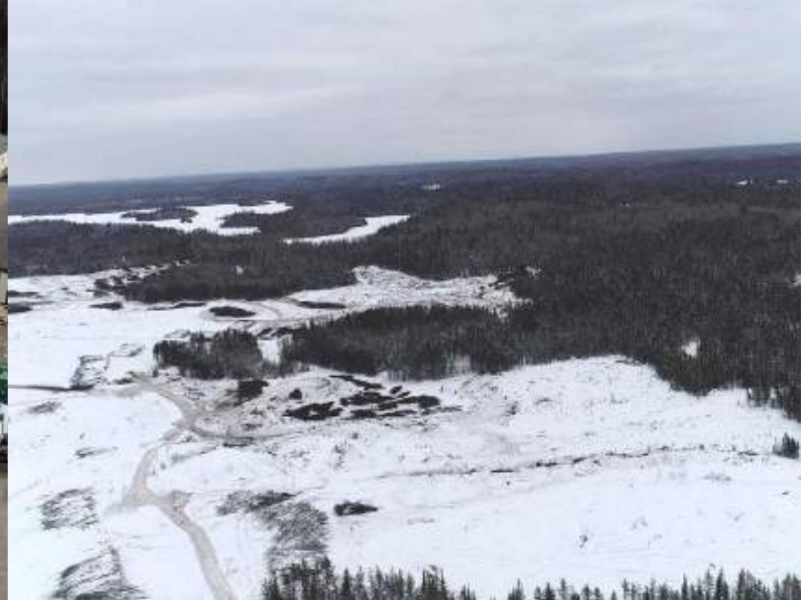
TREE CLEARING – 456 HECTARES COMPLETED
