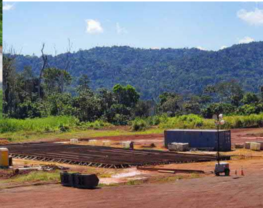
Infrastructure – In Progress
