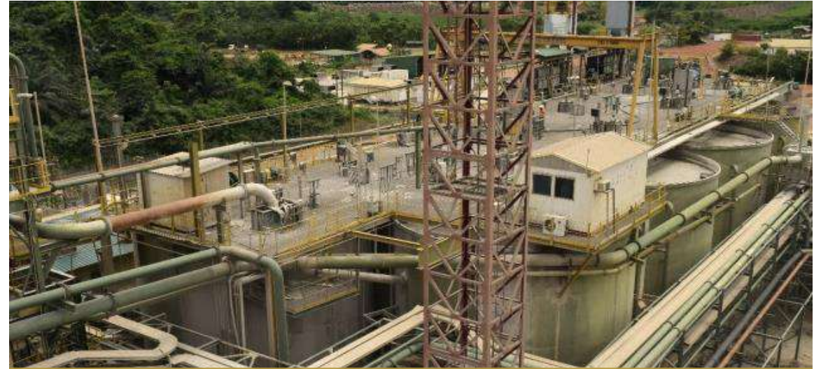
Operational CIL Processing Facility with 3.5 Mtpa Capacity
